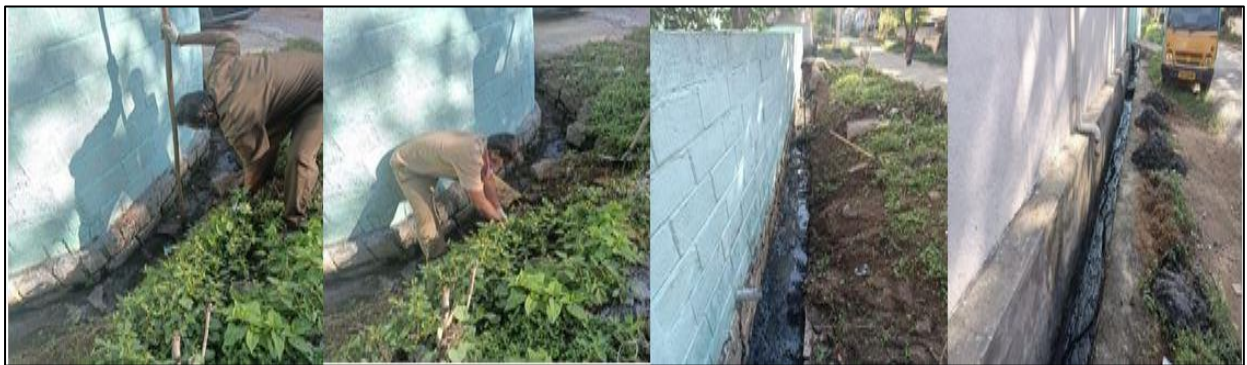
Figure 6. 12: Open Drain Cleaning – Work Process
